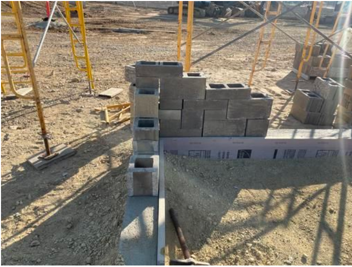
Masonry layout of blocks
