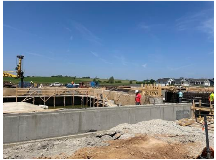
ongoing work on Lap pool
